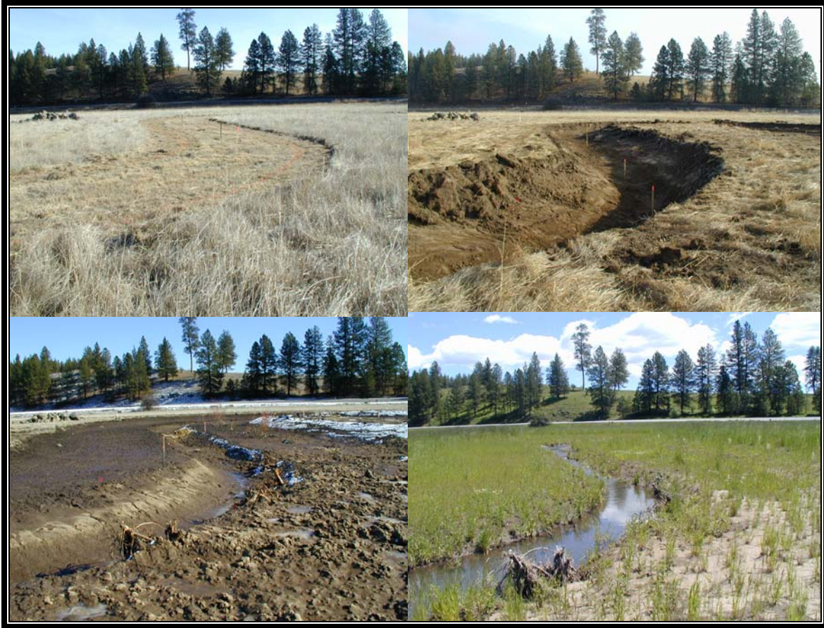
Lower Bear Creek photo sequence taken by ODFW illustrating pre-project 2002, during project, and post project (2003). Note vegetation establishment is just getting underway with one growing season. Initial planting efforts including seeding and installation of sedge/rush plugs and livewhip willow
