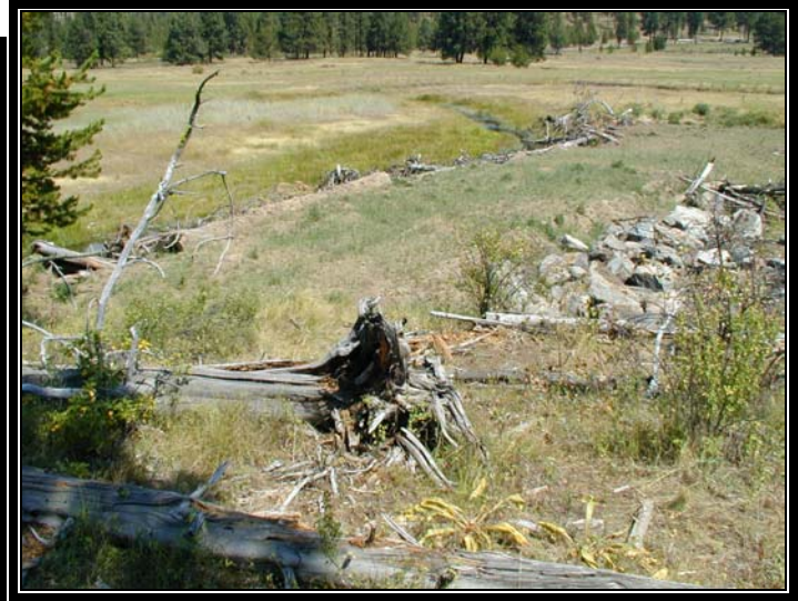
Phase 1 McCoy Creek Restoration Project Diversion Structure (2002)
