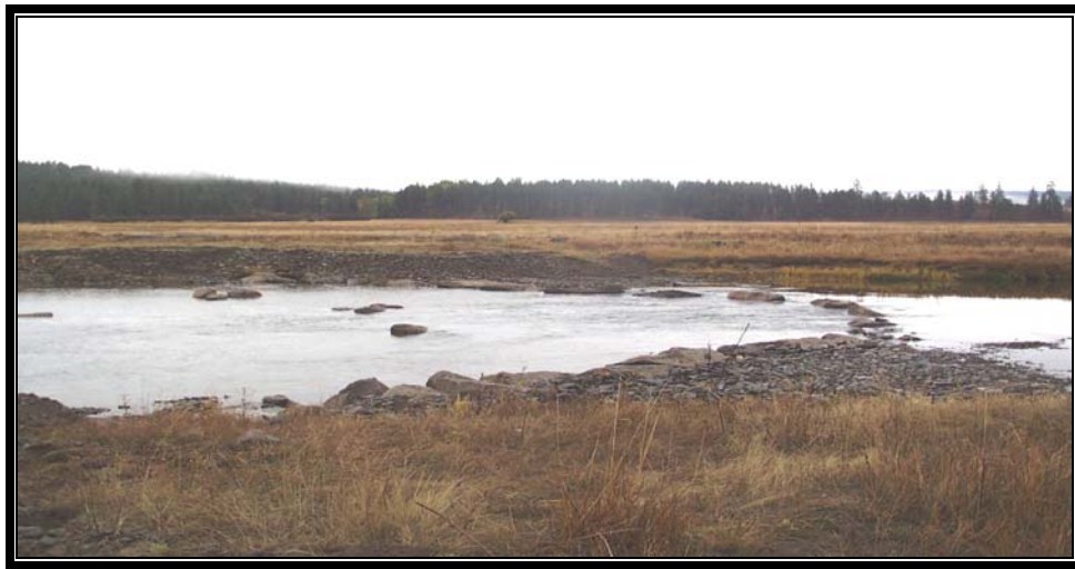
Cross vane rock structure designed to maintain channel grade downstream of the Bear Creek confluence with the Grande Ronde River.
