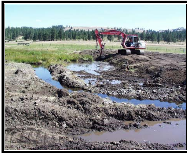
Phase 2 channel excavation and diversion of McCoy Creek into restoration channel
