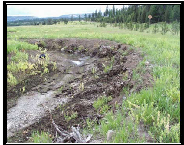
Phase 2 Restoration Channel Construction. October 2001
