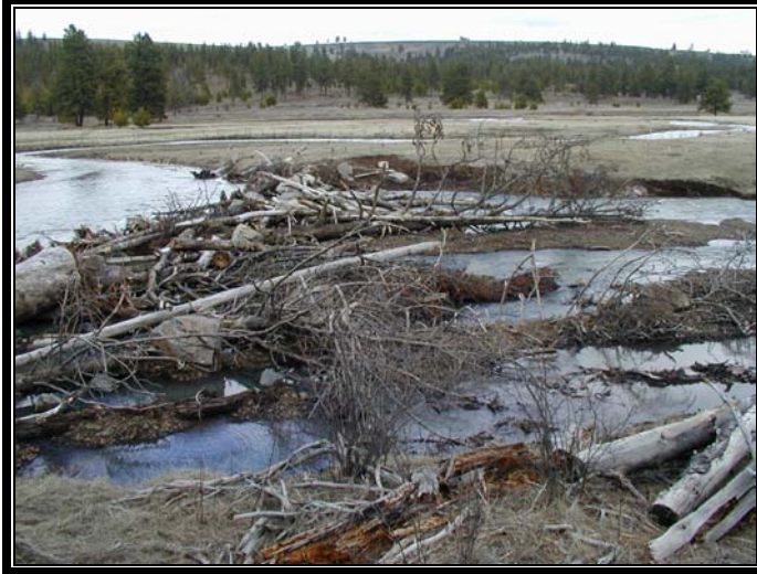
Phase 1 McCoy Creek Restoration Project Diversion Structure (1997)
