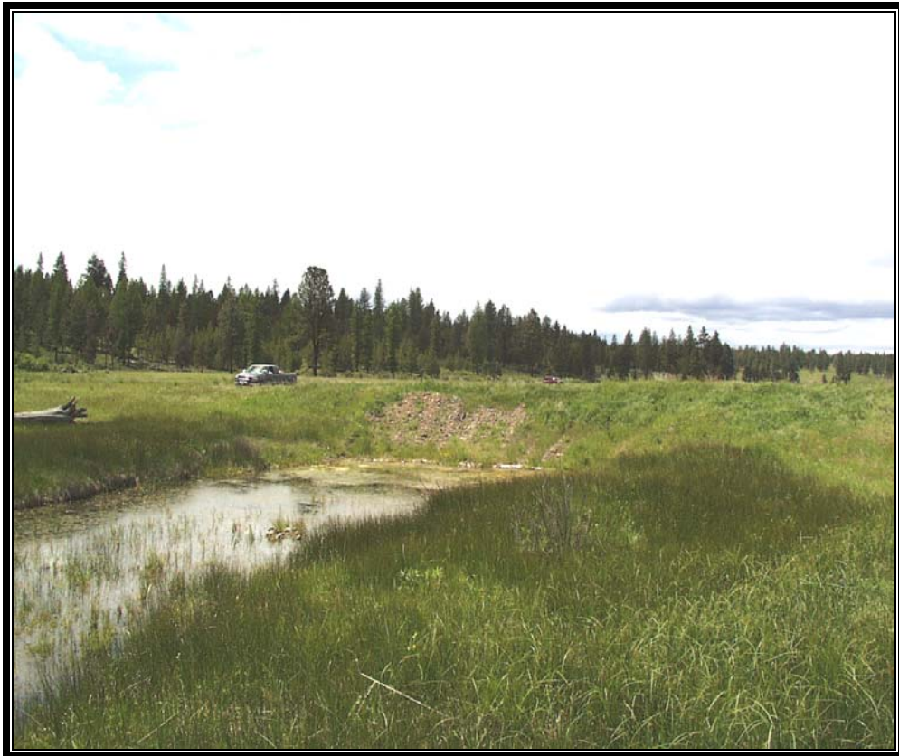
McCoy Meadows 6/02, Photo Point A12-24 (Reclamation activities along pre-project channelized reach. Compacted earthen plug and floodplain pond shaping)
