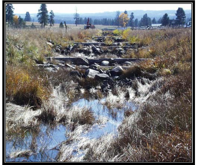
Lower Bear Creek viewing south, upstream. Photo illustrates summer baseflow conditions and lack of fish passage created by log weir structure October 1999.
