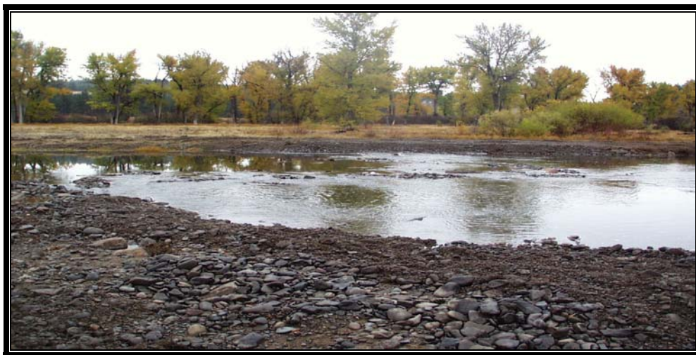
“W” weir installed in Mainstem Grande Ronde River to maintain channel grade, direct thalweg, and improve the width:depth ratio. Structure is located upstream of Jordan Creek confluence.
